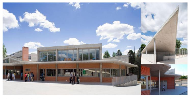
The school is located in the Plaza Duque de Pastrana. It has two storeys below grade and four storeys above grade and is founded on concrete footings. The slabs employed are reinforced solid slabs with maximum spans reaching 10.0m. A post-tensioned 0.36m deep solid slab has been placed to cover a non-continuous 13.0m span. In the dining room areas the roof employs sloping concrete slabs.
